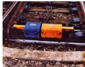
Figure 6 – Train Operated Points
