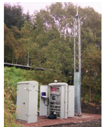
Figure 15 – Typical TRCU Installation
