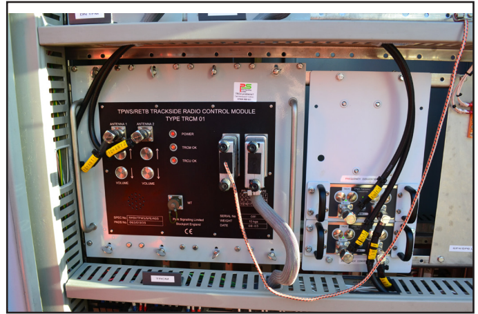
Figure 13 – Trackside Radio Control Module (TRCM)
