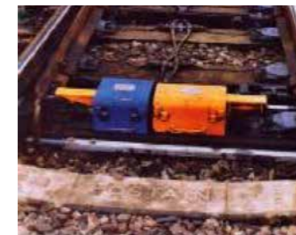
Figure 6 - Train Operated Points
