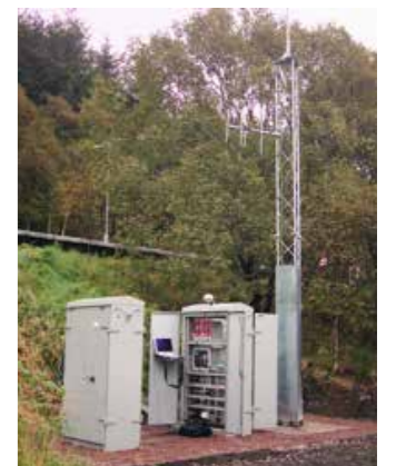
Figure 15 – Typical TRCU Installation
