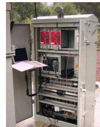
Figure 14 – Typical TRCM Installation
